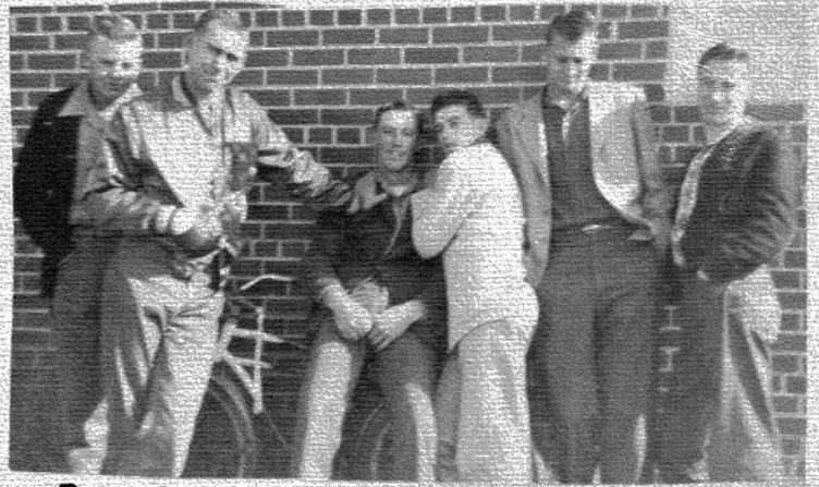
PROPS ARE DANGEROUS
