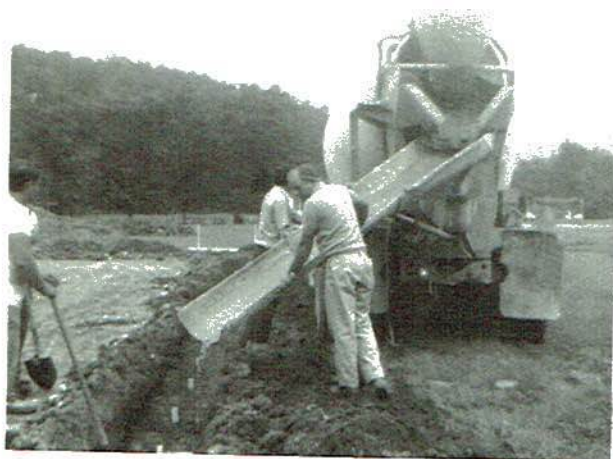
Foundation is started.
