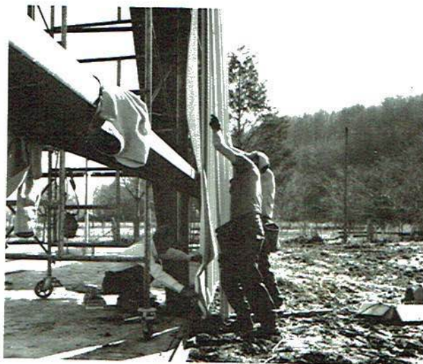
The Beams go up.
