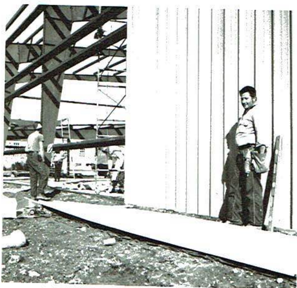
The first wall rises.
