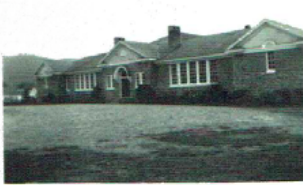
Paint Rock Valley High School Princeton, Alabama
