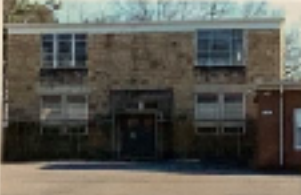
Photo of current Flat Rock High School Administration Building as seen in 2000. 13 year construction. In use since 1997 with newly restored offices.
