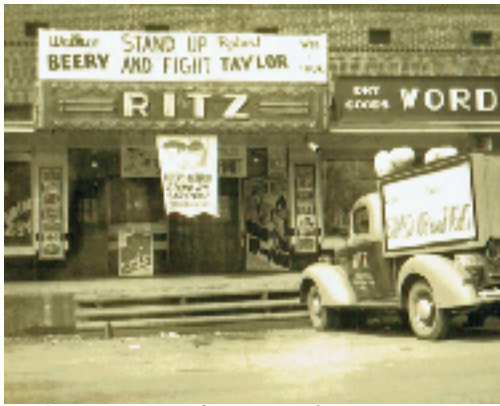
Early 1940s picture, showing wooden stair access to elevated sidewalk.
