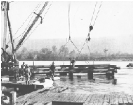
L to R., construction of the Widows Creek bar and dam; Men setting the last crib; and construction of the lock. Photos owned by Marion Lloyd.
