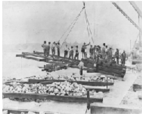
L to R., construction of the Widows Creek bar and dam; Men setting the last crib; and construction of the lock. Photos owned by Marion Lloyd.
