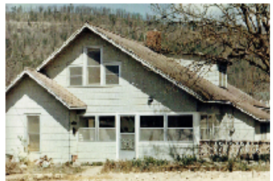
The Cothron boarding house at 212A Elm Street.
