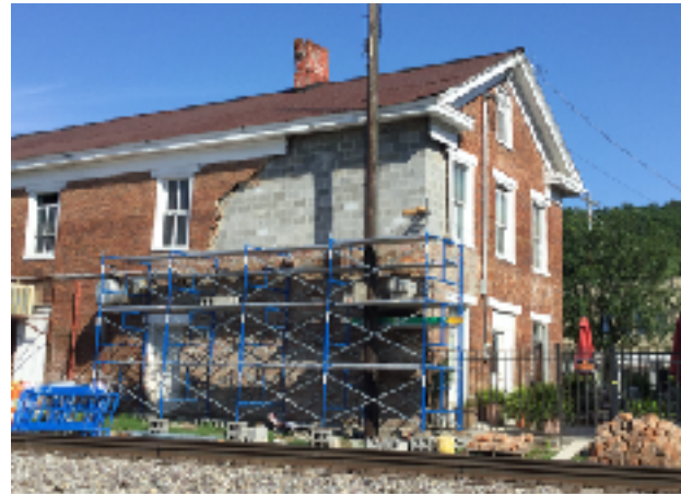
June 5, 2018 with repairs in progress
