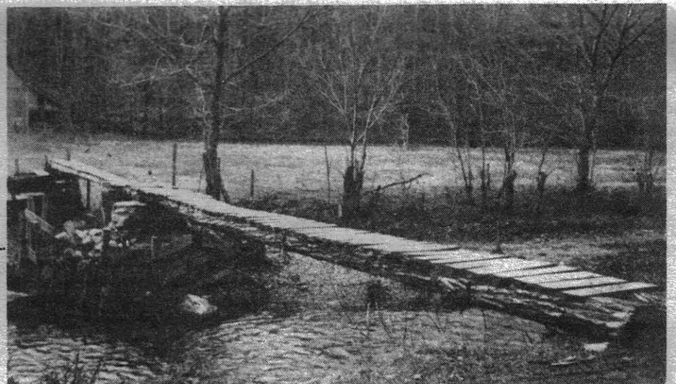
A log bridge over Larkin's Fork Creek
